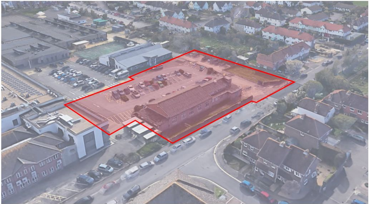
Aerial View of the site, looking south west
